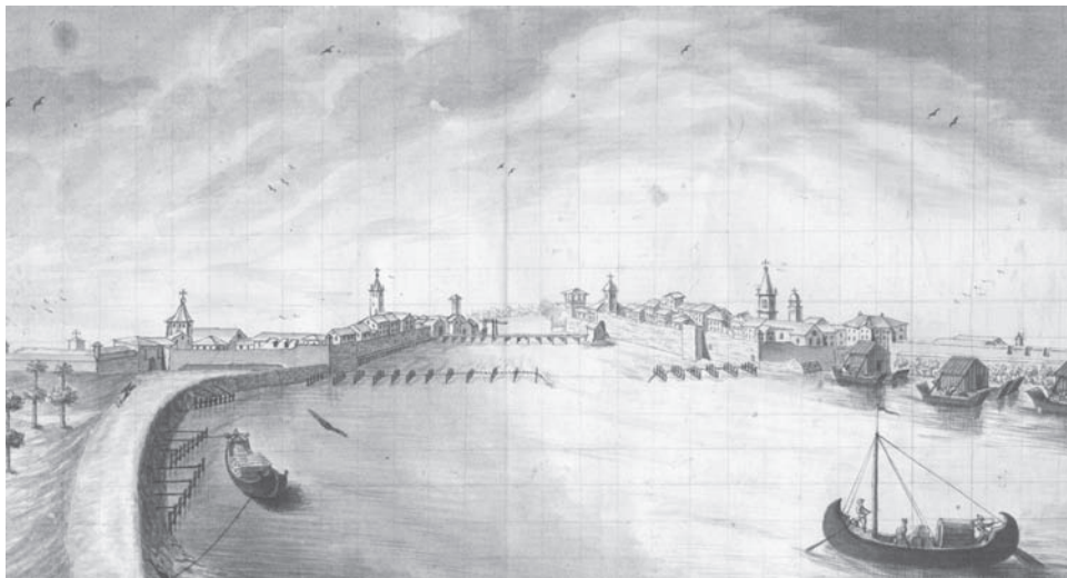
Figure 7: The Adige enters the fortified town of Legnago-Porto (eighteenth century). Left: the towing path; the wooden groins (pennelli) protecting the levee. Beyond lies Porto. Right: floating mills and Legnago. Across the river, the chain (lowered) and further downstream, the wooden bridge. (Veduta di Legnago, BCVR, Stampe 2.a.226, foglio 32)
